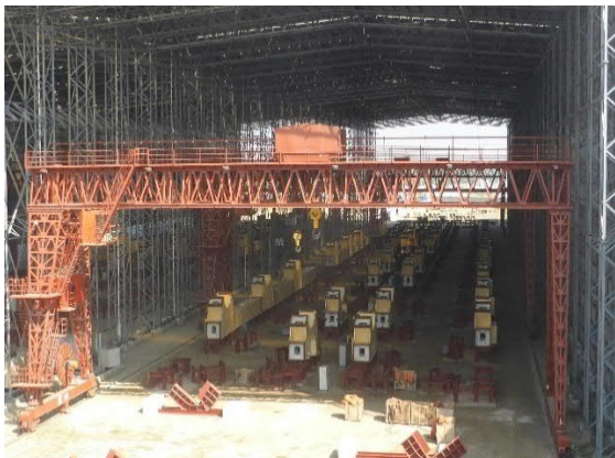
Figure 9. Site pre-assembly at Mawa
