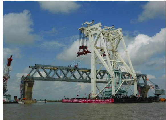
Figure 11. Truss Erection
