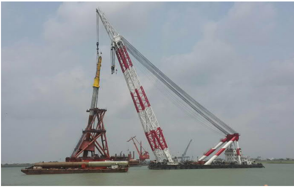
Figure 4. Guide frame and foundation pile driving
