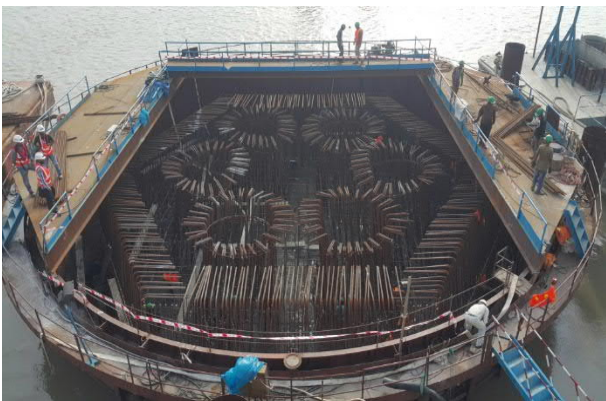
Figure 5. Cofferdam and Pile Cap Reinforcement
