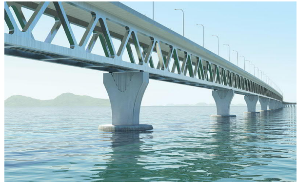
Figure 6. Schematic of deck, truss and pier.
